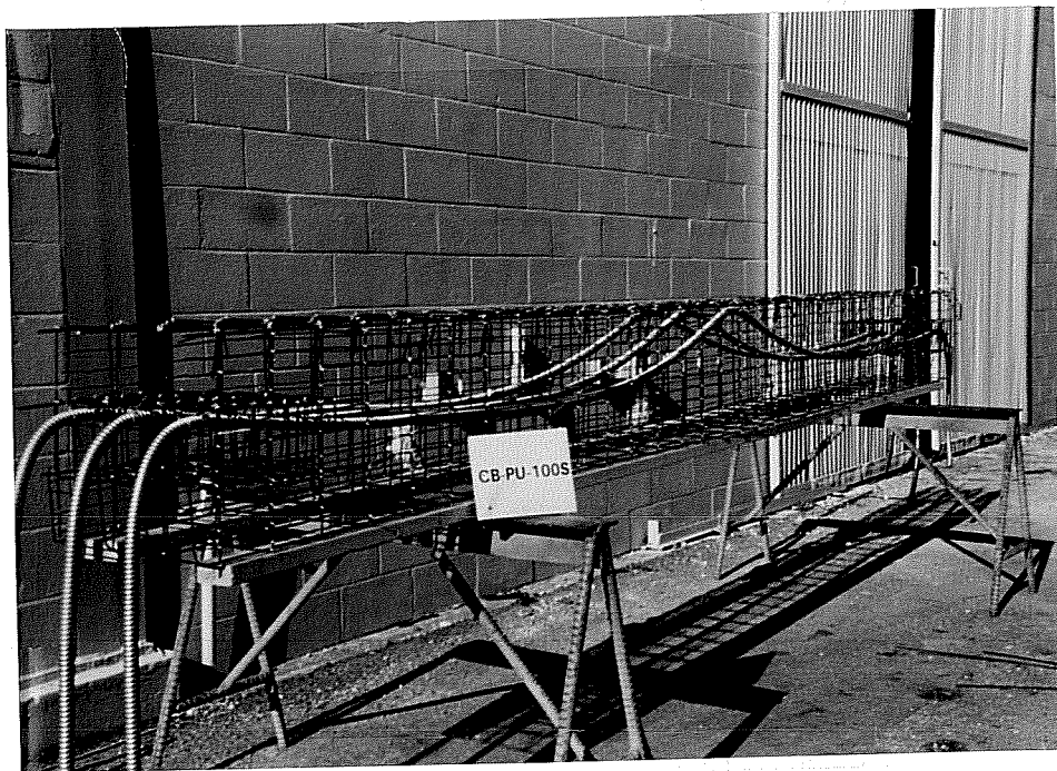
Figure 3.22 Fabrication of Reinforcing Cage
