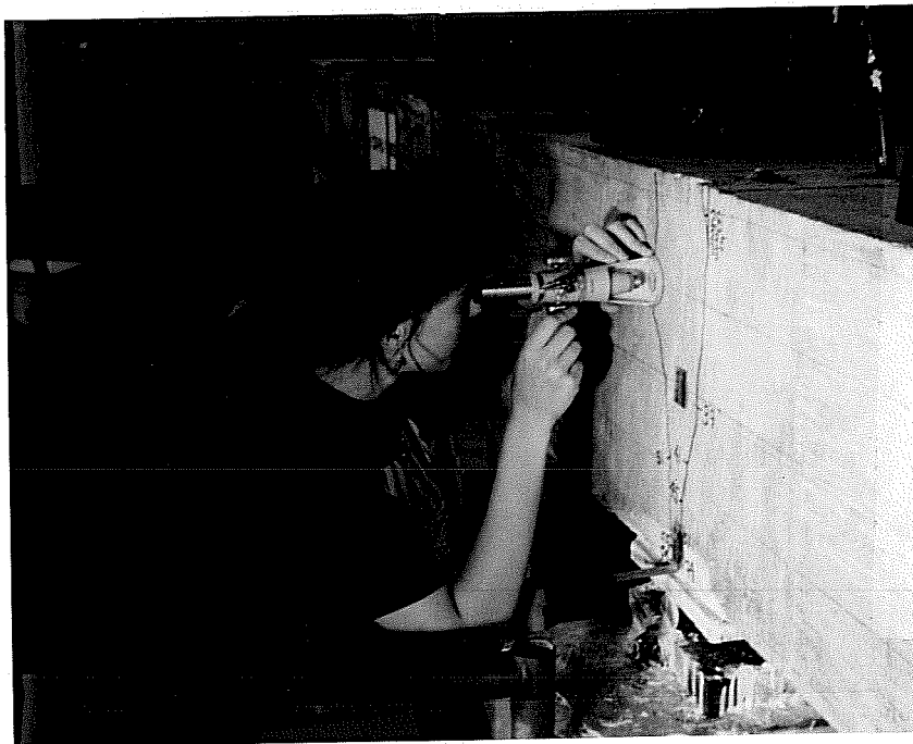
Figure 3.33 Measuring of Crack Widths with an Optical Crack Monitor
